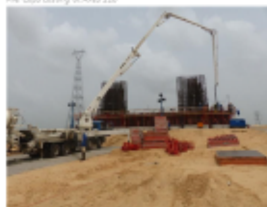
Area 100 - casting driven piles
