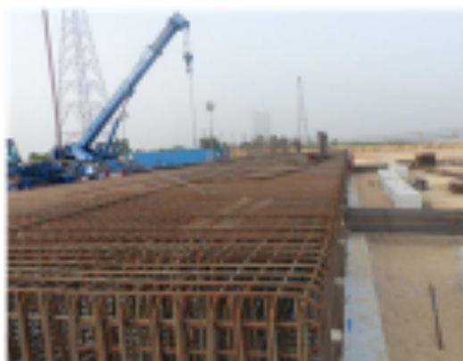
Area 100 - Fixing pile cap reinforcement - completed
