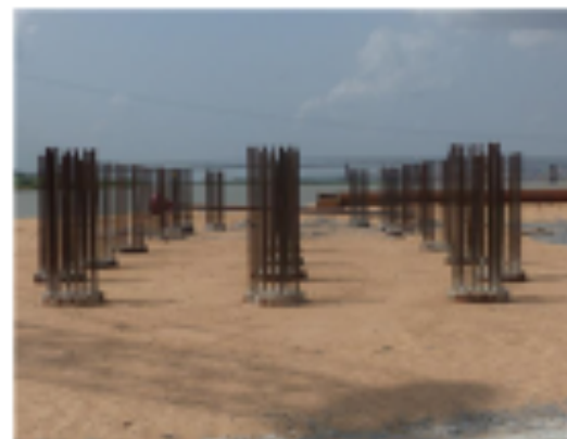
Area 100 - casting driven piles
