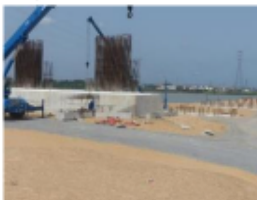
Area 100 - Fixing pile cap reinforcement - completed
