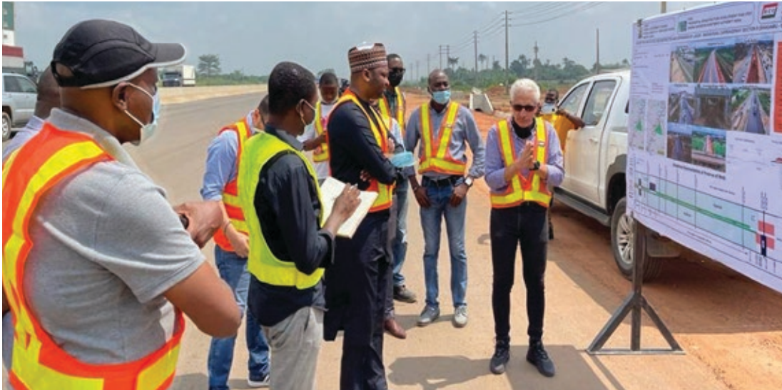
NED, Sir Babatunde Sobamowo, KJW (far left) and ED, Mr. Aminu Umar-Sadiq (centre) with RCC Project Manager on the Lagos-Ibadan Expressway during a site inspection.
