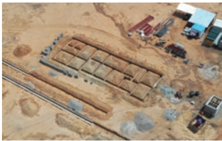
Kano Solar Project earth works.
