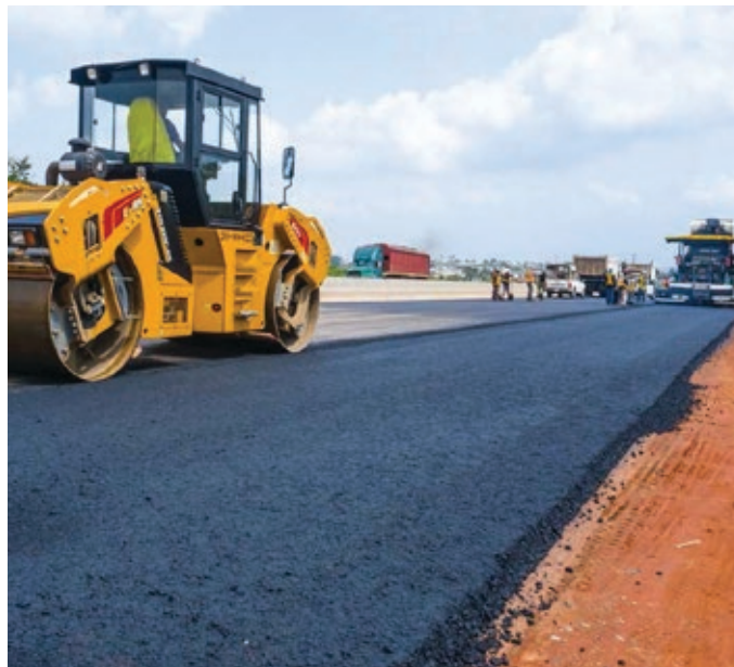
Laying asphaltic base course for the Lagos-Ibadan Express.
