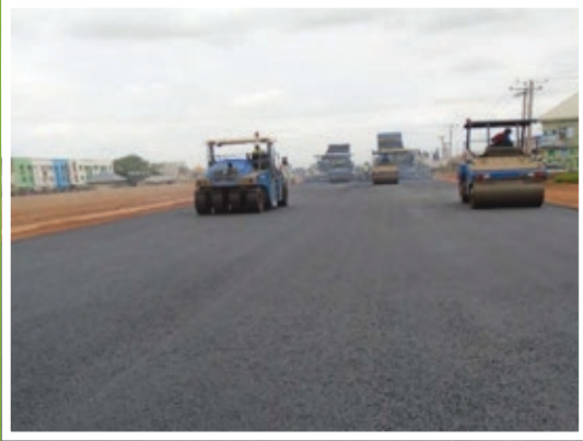
Groundworks on the Abuja-Kano Road Project.
