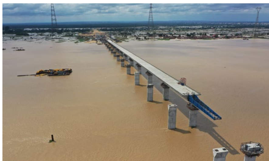
Second Niger Bridge.
