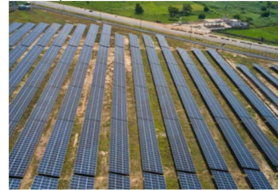
10MW Solar Farm in Kumbotso Local Government Area of Kano State
