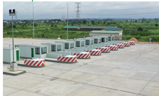
Toll booths at the Second Niger Bridge
