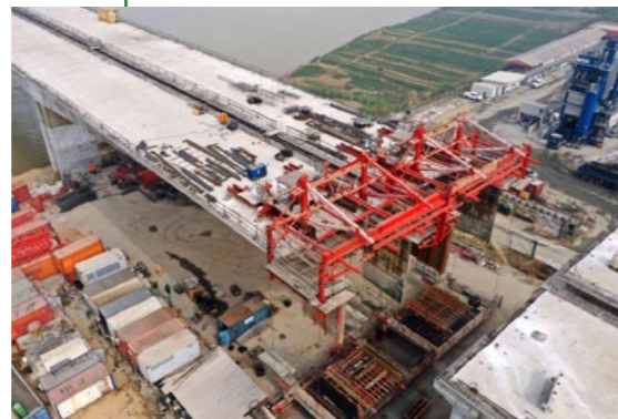
Second Niger Bridge under construction
