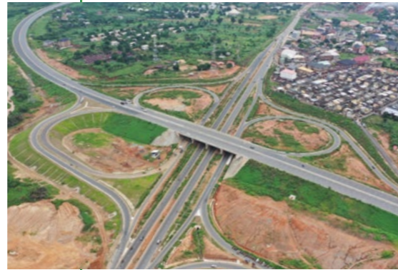
The Owerri interchange constructed under the PIDF
