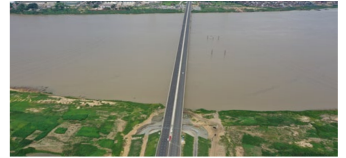
Second Niger Bridge constructed under the PIDF
